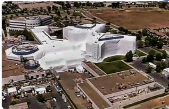
12 Storey hospital in the USA wrapped in plastic for chlorine dioxide gas disinfection,
